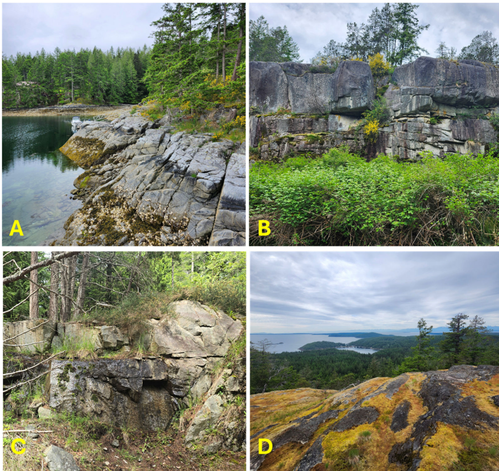
Figure 9. Granitic bedrock outcrops on Cortes Island exhibit large blocky fractures that can store and transmit groundwater. A) In coastal areas such as Cortes Bay, wells that intercept fractures connected to coastal zones may draw in brackish (mixed) or saline water. B) Large vertical and horizontal fractures in outcrop near Manson's Landing. C) Water seepage from outcrop near the Whaletown ferry terminal. D) Easter Bluff looking south: In upland areas, the bedrock is overlain by a thin layer of soil or sediments promoting more rapid runoff and increasing vulnerability to contaminants introduced at the surface .
