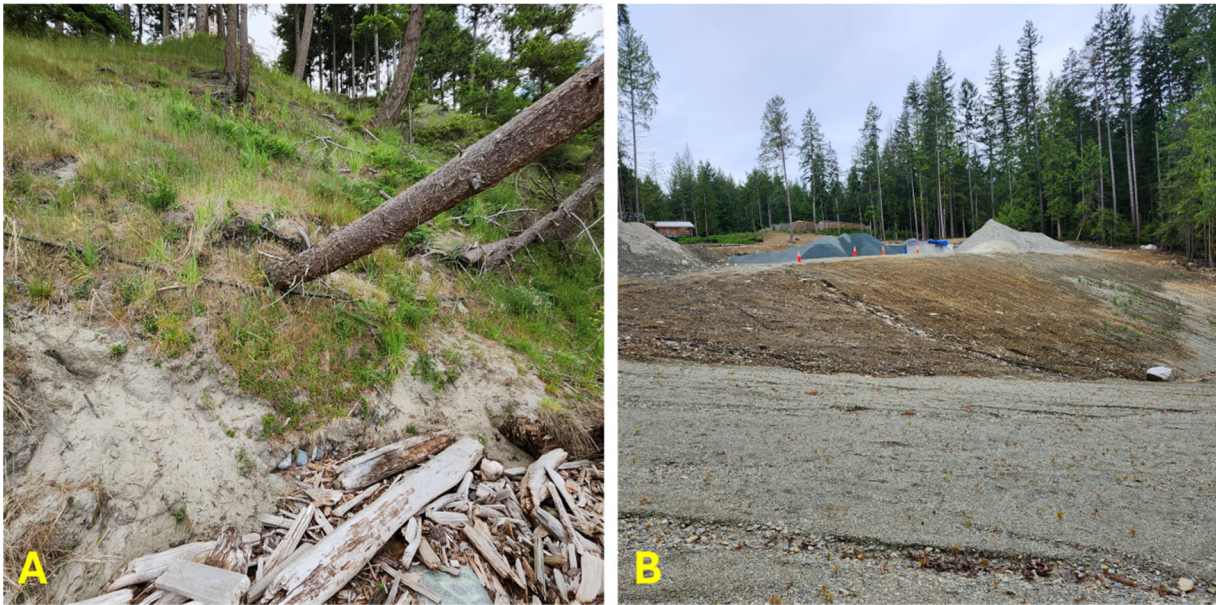
Figure 8. A) Unstable coastal bluff southeast of Manson's Landing shows silt and fine sand layers which overly the principal aquifer AQ841. B) Land clearing near Squirrel Cove has exposed a locally thick deposit of gravel and sand which overlies and forms a previously unmapped unconsolidated aquifer in this area.
