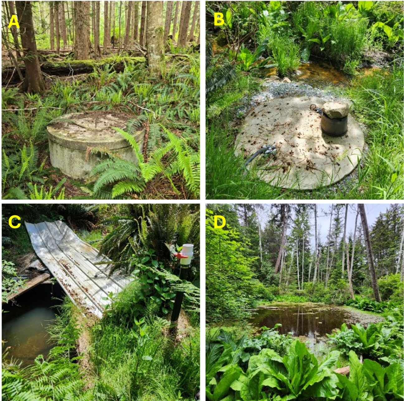
Figure 4. Spring water sources can have the appearance of A) shallow dug well, B) stilling well adjacent to a stream, or C) small dugouts. D) Natural wetland areas may indicate areas of spring discharge or be associated with perched water systems. Spring water sources are shallow and vulnerable to contamination and seasonal decline in water availability.
