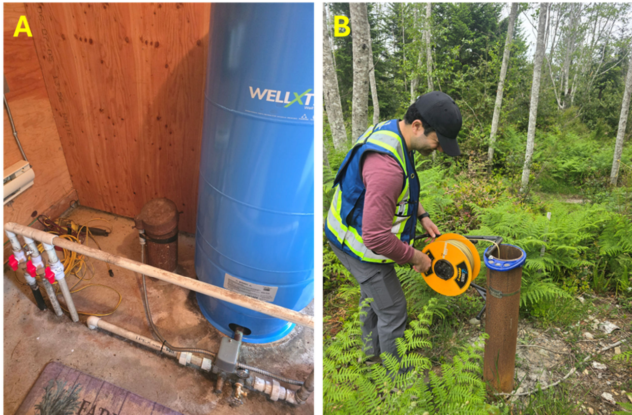
Figure 6. Example of drilled wells observed on Cortes Island. A) Domestic well in a pump house, and B) measuring groundwater level at the Rainbow Ridge development well.
